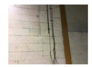
Location: Elevation 5 Condition: Very poor Decorative Condition: N/a Comments: Redundant cabling
