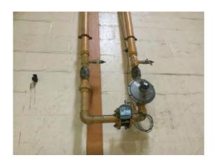
Location: Elevation 4 Condition: Fair Decorative Condition: Poor Comments: Gas meter - not tested, soiled pipework
