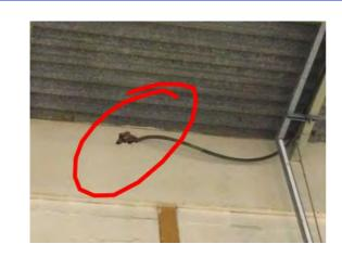
Location: Elevation 5 Condition: Poor Decorative Condition: N/a Comments: Infilled service penetration
