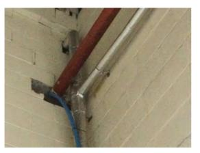
Location: Elevation 3 Condition: Poor Decorative Condition: N/a Comments: Service penetrations not fire stopped
