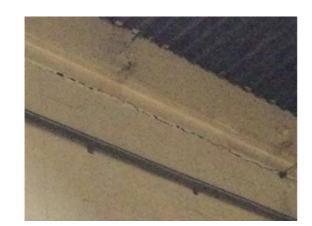
Location: Elevation 4 Condition: N/a Decorative Condition: N/a Comments: Cracking under the ring beam at high level
