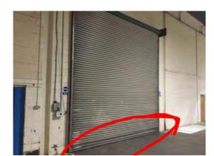
Location: Elevation 2 Condition: Fair Decorative Condition: Poor Comments: Soiled shutter door, impact damage at low level
