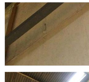
Location: Elevation 5 Condition: Fair Decorative Condition: Very poor Comments: Rippled and lifting joint tape to the partition wall
