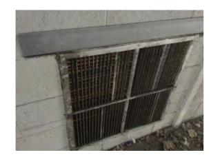
Location: Elevation 1 Condition: Poor Decorative Condition: N/a Comments: Aged, corroded and soiled vent
