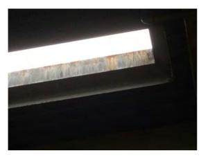
Location: Bay 1 Condition: Poor Decorative Condition: N/a Comments: Corrosion around the rooflight
