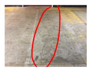
Location: Bay 9 Condition: Poor Decorative Condition: N/a Comments: Heavy cracking running towards the exit door
