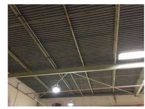
Location: Bay 3 Condition: Fair Decorative Condition: Poor Comments: Roof cladding is heavily soiled, steelwork affected by surface corrosion
