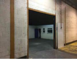
Location: Elevation 5 Condition: Very poor Decorative Condition: Poor Comments: Soiled decorations, door missing
