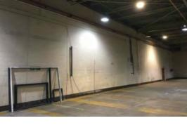
Location: Elevation 3 Condition: Poor Decorative Condition: N/a Comments: Corroded barrier around the water main
