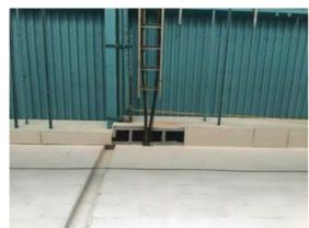
Location: Elevation 1 Condition: Poor Decorative Condition: N/a Comments: Missing section of fire cladding
