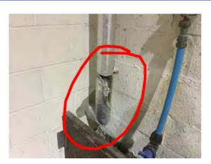
Location: Elevation 3 Condition: Poor Decorative Condition: N/a Comments: Damaged pipe lagging
