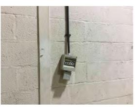
Location: Elevation 3 Condition: Poor Decorative Condition: N/a Comments: Displaced gas heater control
