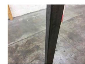
Location: Office 1 Condition: N/a Decorative Condition: Poor Comments: Corroded steel support post
