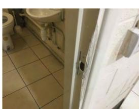
Location: Dis WC Condition: Poor Decorative Condition: Poor Comments: Damage door frame
