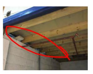
Location: Storage area Condition: Poor Decorative Condition: N/a Comments: Exposed timber structure - lack of fire stopping
