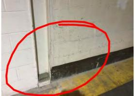
Condition: Fair Decorative Condition: Poor Comments: Minor impact damage to the column to the left of the double doors
