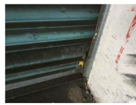
Location: Elevation 1 Condition: Fair Decorative Condition: Poor Comments: Damage to lower right corner
