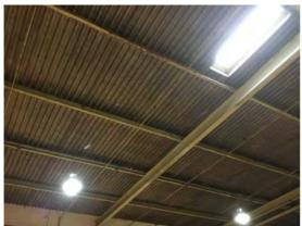
Location: Bay 1 Condition: Fair Decorative Condition: Poor Comments: Roof cladding is heavily soiled, steelwork affected by surface corrosion
