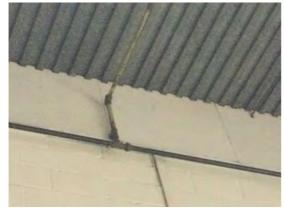
Location: Elevation 2 Condition: Poor Decorative Condition: N/a Comments: Corroding, redundant pipework
