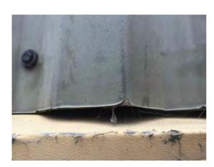
Location: East elevation Condition: Poor Decorative Condition: N/a Comments: The cladding is affected by cut edge corrosion
