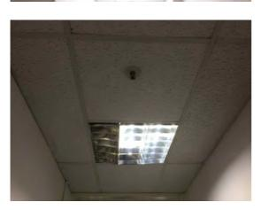
Location: Corridor 1 Condition: Poor Decorative Condition: N/a Comments: Defective lamp and displaced light diffuser
