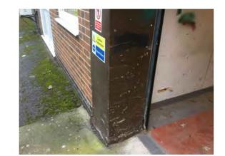
Location: East elevation Condition: Poor Decorative Condition: N/a Comments: Scuffed left hand reveal flashing
