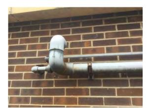
Location: Outbuilding Condition: N/a Decorative Condition: N/a Comments: Corroded brackets to the vent pipe
