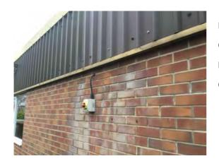
Location: West elevation Condition: Poor Decorative Condition: N/a Comments: Water stained brickwork
