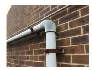
Location: Outbuilding Condition: Poor Decorative Condition: N/a Comments: Corroding vent pipe brackets
