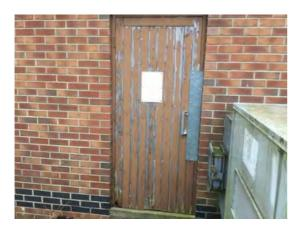
Location: West elevation Condition: Poor Decorative Condition: Poor Comments: Exit door - peeling paintwork, decay at low level
