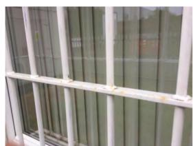
Location: West elevation Condition: Fair Decorative Condition: Poor Comments: Corroded security bars
