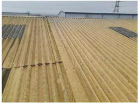
Location: Roof Condition: Poor Decorative Condition: N/a Comments: Flashing between the roof sheets
