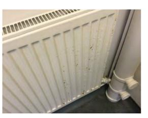
Location: Male WC 2 Condition: Poor Decorative Condition: Poor Comments: Corroded radiator, blistered paint finish
