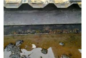
Location: Roof Condition: Poor Decorative Condition: N/a Comments: Corroded west gutter and standing water
