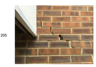
Location: South elevation Condition: Poor Decorative Condition: N/a Comments: Structural cracking
