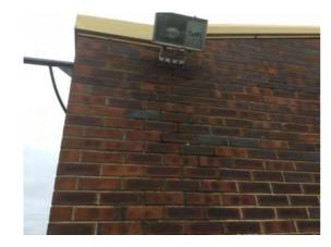
Location: South elevation Condition: Poor Decorative Condition: N/a Comments: Weathered pointing
