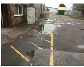
Location: East access road Condition: Poor Decorative Condition: N/a Comments: Undulating road surface and ponding water
