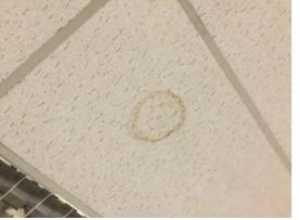
Condition: Poor Decorative Condition: N/a Comments: Sporadic water stained ceiling tiles due to roof leaks
