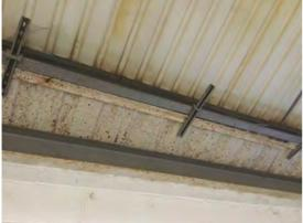
Condition: Poor Decorative Condition: N/a Comments: Corrosion to the cladding and underside of the gutters
