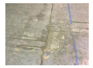
Location: Main Warehouse Condition: Poor Decorative Condition: Poor Comments: Unevenness and patch repairs
