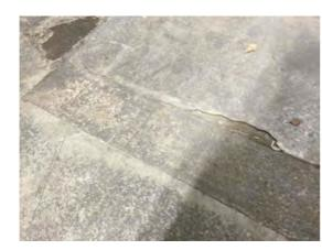
Location: East Warehouse Condition: Poor Decorative Condition: N/a Comments: Screed repair, delaminating surface finish
