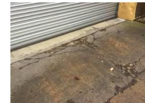
Condition: Poor Decorative Condition: N/a Comments: Cracked concrete forward of the loading doors
