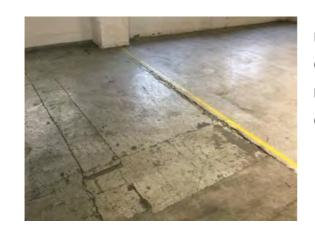
Location: Main Warehouse Condition: Poor Decorative Condition: Poor Comments: Cracked and frayed bay joints
