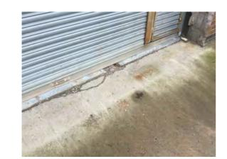
Location: East access road Condition: Fair Decorative Condition: N/a Comments: Cracked concrete to the loading bay threshold
