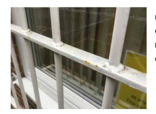
Location: East elevation Condition: Fair Decorative Condition: Poor Comments: Light corrosion affecting the window bars
