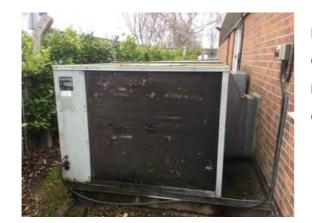
Location: Western boundary and verge Condition: Very poor Decorative Condition: N/a Comments: Redundant AC condenser/ air handling unit
