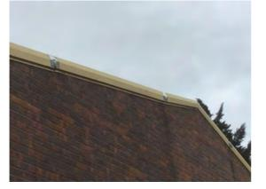
Location: South elevation Condition: Poor Decorative Condition: N/a Comments: Verge cappings - solar faded and joints taped
