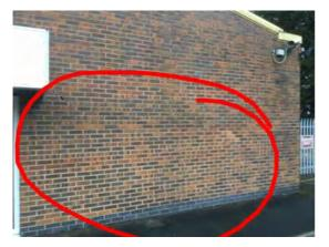
Location: South elevation Condition: Poor Decorative Condition: N/a Comments: Area of wall affected by structural movement
