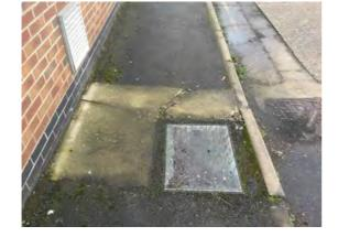
Location: East access road Condition: Poor Decorative Condition: N/a Comments: Cracking around a galvanised drain cover
