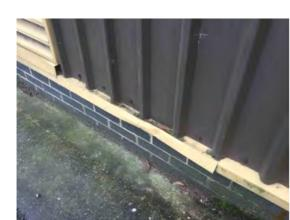
Location: North elevation Condition: Poor Decorative Condition: N/a Comments: Displaced and indented sill trim
