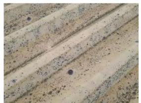
Location: Roof Condition: Poor Decorative Condition: N/a Comments: Corroding fixings and missing caps
