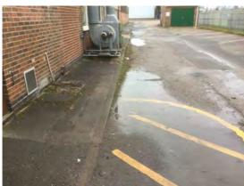
Location: East access road Condition: Poor Decorative Condition: N/a Comments: Ponding water and undulations
