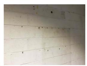
Location: East Warehouse Condition: N/a Decorative Condition: Poor Comments: Many redundant fixing holes in the blockwork
