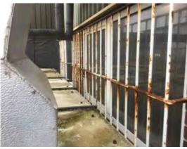
Location: West elevation Condition: Poor Decorative Condition: Poor Comments: Corroded security bars
