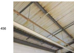
Location: Main Warehouse Condition: Poor Decorative Condition: N/a Comments: Corrosion affecting cladding along the east pitch
