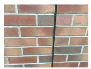
Location: West elevation Condition: Poor Decorative Condition: N/a Comments: No mastic provided to the expansion joints
