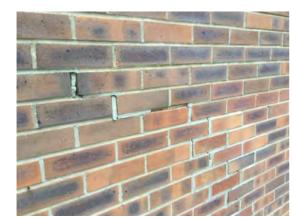
Location: South elevation Condition: Poor Decorative Condition: N/a Comments: Stepped structural cracking
