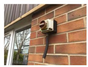
Location: West elevation Condition: Very poor Decorative Condition: N/a Comments: Disconnected power isolator
