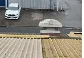
Location: Roof Condition: Poor Decorative Condition: N/a Comments: Indented edge capping - west pitch
