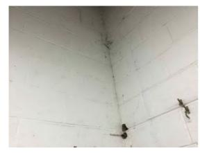
Location: Boiler Room Condition: Fair Decorative Condition: Poor Comments: Soiled paintwork, hairline cracking
