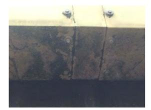
Location: North elevation Condition: Poor Decorative Condition: N/a Comments: Leaky gutter joints, corroding and silted gutter
