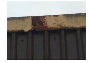
Location: East elevation Condition: Poor Decorative Condition: N/a Comments: Badly corroded section of metal facia
