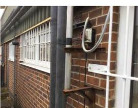
Location: West elevation Condition: Poor Decorative Condition: N/a Comments: Corroding brackets
