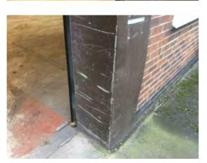
Location: East elevation Condition: Poor Decorative Condition: N/a Comments: Scuffed right hand reveal flashing
