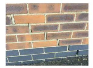
Location: South elevation Condition: Poor Decorative Condition: N/a Comments: Stepped cracking
