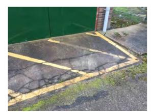
Location: East access road Condition: Poor Decorative Condition: N/a Comments: Cracked ramp to the outbuilding
