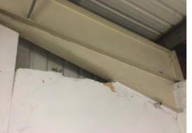
Condition: Poor Decorative Condition: N/a Comments: Missing section of blockwork below a steel portal haunch
