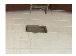
Location: East Warehouse Condition: Poor Decorative Condition: N/a Comments: Missing block - lack of fire stopping
