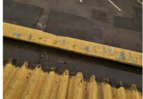
Decorative Condition: N/a Comments: Corroding gutter - indented edge capping to the east pitch
