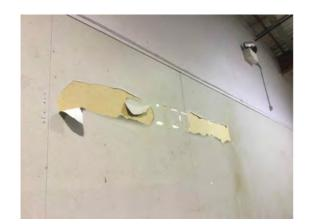
Location: East Warehouse Condition: Poor Decorative Condition: Poor Comments: Delaminating paper finish to the partition wall
