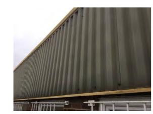
Location: West elevation Condition: Fair Decorative Condition: Poor Comments: Solar faded cladding - perished fixing caps
