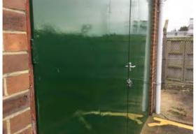
Condition: Poor Decorative Condition: N/a Comments: Doors have been lined in plywood, doors assumed to be decayed
