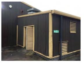
Location: North elevation Condition: Poor Decorative Condition: N/a Comments: Indented cladding and trims
