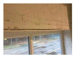
Location: East Warehouse Condition: N/a Decorative Condition: N/a Comments: Cracking above the window head
