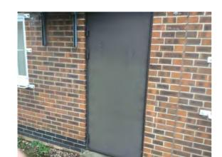
Location: West elevation Condition: Fair Decorative Condition: Poor Comments: Solar faded exit door
