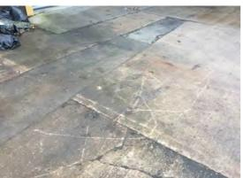
Location: Yard Condition: Poor Decorative Condition: N/a Comments: Cracked, scuffed and stained concrete
