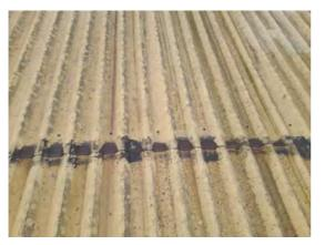
Location: Roof Condition: Poor Decorative Condition: N/a Comments: Heavy corrosion to the overlap joints
