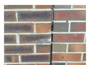
Location: East elevation Condition: Poor Decorative Condition: N/a Comments: Missing mastic to the expansion joints
